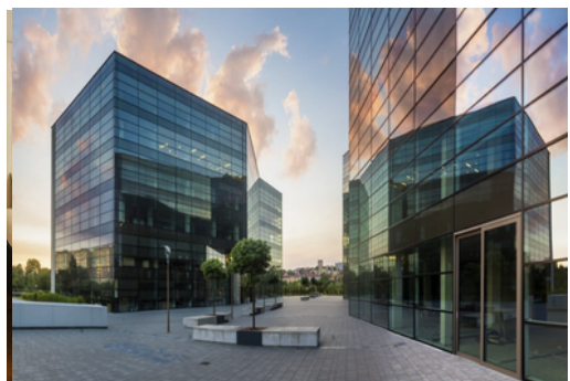
COMMERCIAL COMPLEX , ANUJGLOBAL HOMES
